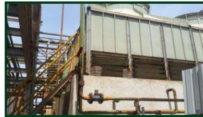
Cooling tower make up
