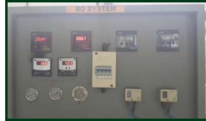
WTP –Ro plant (process )
