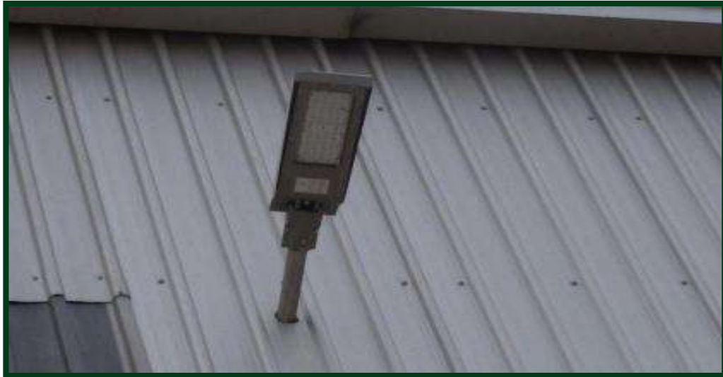
LED Lights(100 Watts) are being used in place of metal halide lamps
