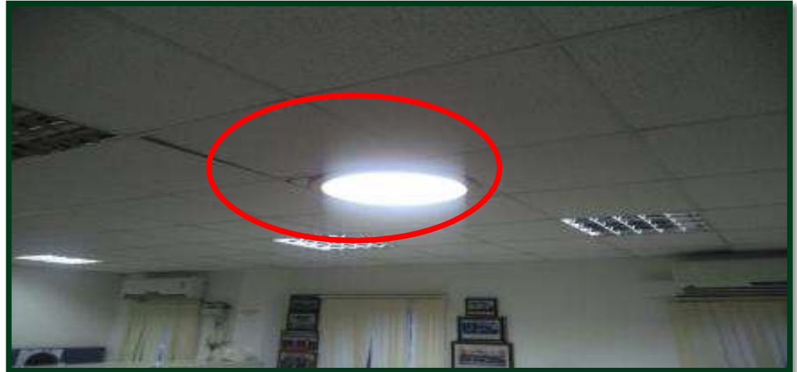
Solar Light pipes in our office
