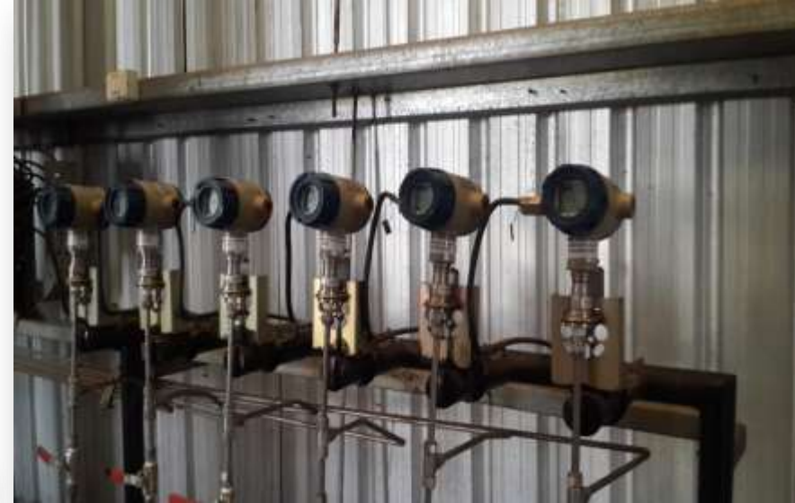
Online Pressure transmitter at PRS station
