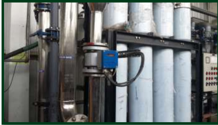
WTP – ultra filtration plant
