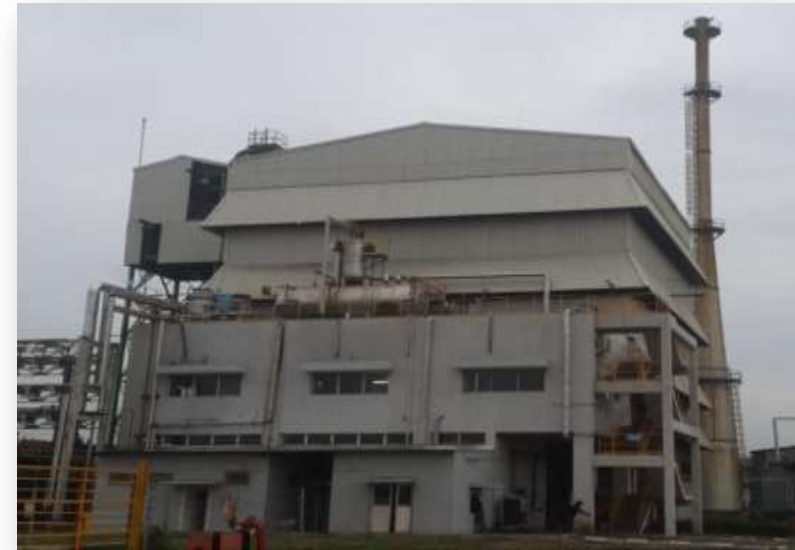
AFBC Coal Boiler IPO Oil Fired Boiler
