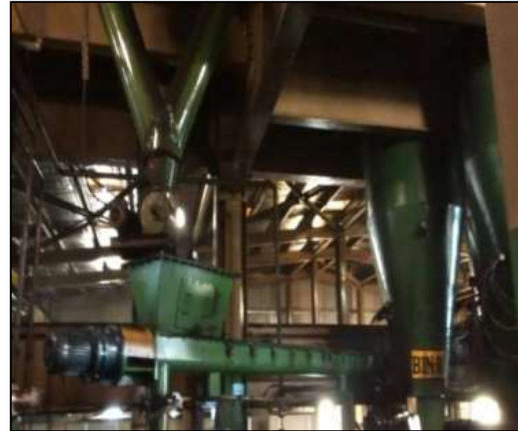
DUST COLLECTOR SYSTEM
